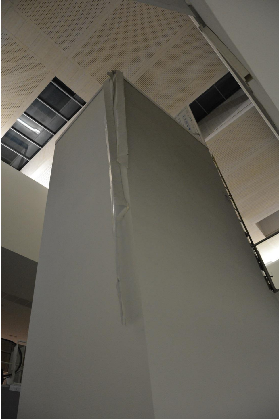
The lift tower in the hospital hall.
