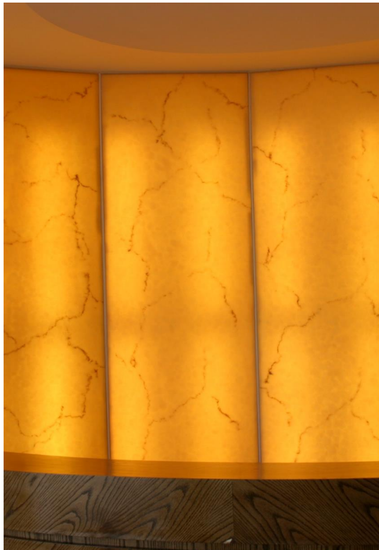
Backlighting with fluorescent tubes: missing homogeneity.
