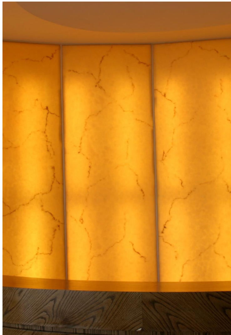
Backlighting with fluorescent tubes: missing homogeneity.
